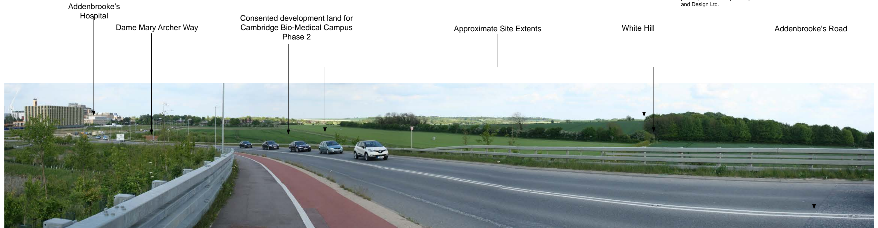
PH T VIEWP INT 3: View east from rail bridge, Addenbrooke's Road
